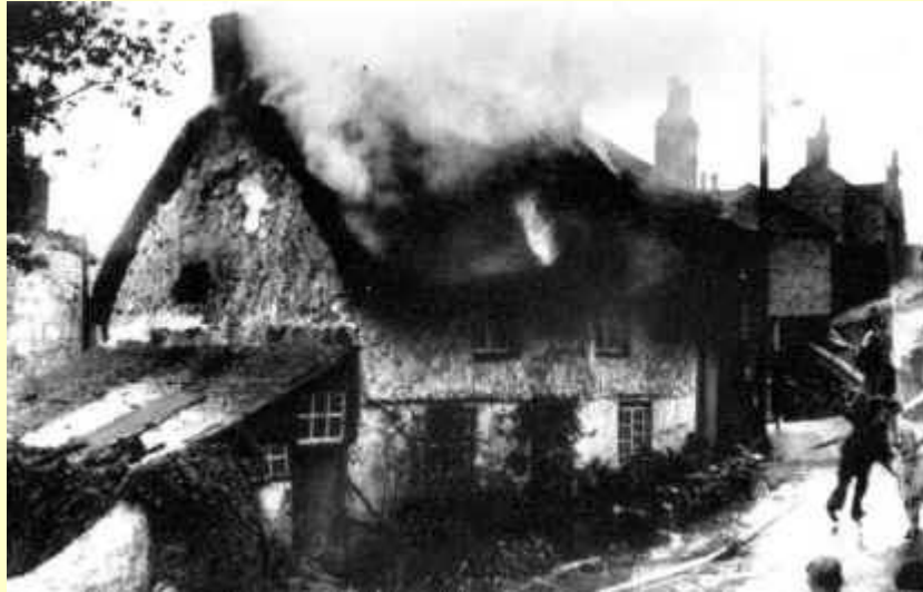
The Last Thatched Cottage in Newlyn on Church Lane
